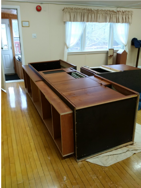
Installing lift Section
