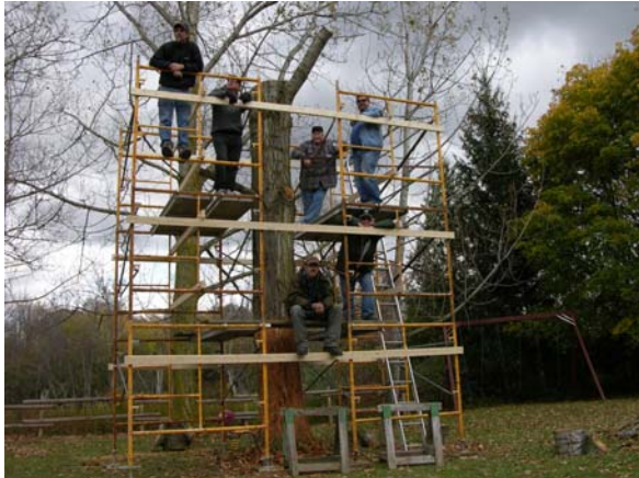
Scaffolding set up crew
