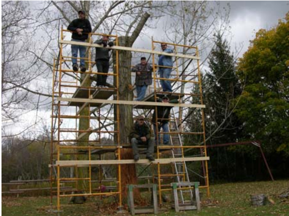
Scaffolding set up crew
